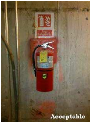
Fire extinguisher in a construction site.
